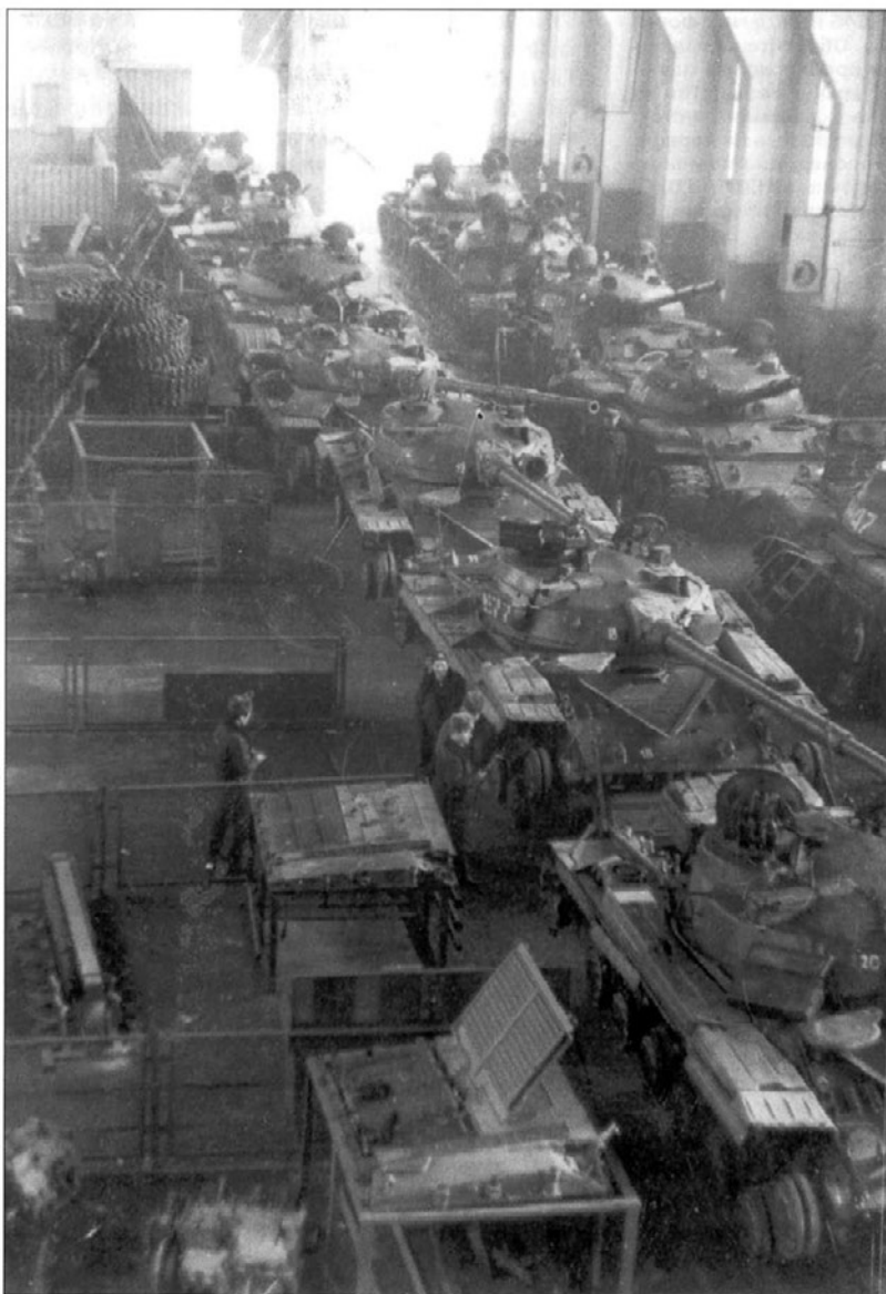
Цех 1-й роты ОРВБ 2 ГвТА. Слева колонна ремонтируемых Т-64А, справа – Т-62. ГСВГ, 1983 г. Фото М. Чобитка. A workshop of the 1st company, reconstruction and repair independent battalion, 2nd guards tank army. To the left is a column of reparable T-64A tanks, to the right – T-62 tanks, Soviet Forces Group in Germany, 1983.
